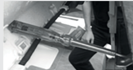
Small connection space
