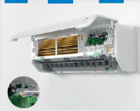
Open the electrical panel and disconnect the fan motor and the louver motor
