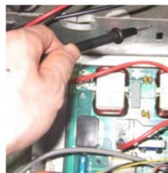
Figure 4-4.5: Measuring resistances between compressor terminals and ground
