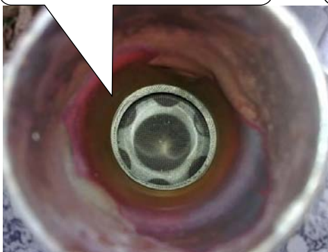
A clean filter (on the suction pipe of the system)
